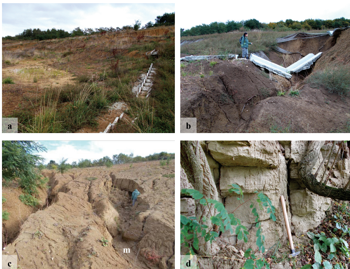
Figure 2. Outcrop photographs in the Bucium Hill area (original, September 2017). a, b) Landslides in the clays from the eastern part of the cutting slope; destroyed drainage works and textile net are seen. c) Gullies in the clayey sands from the western part of the cutting slope, with marls (m) on the bottom of the deep gullies. d) Sistematically fissures on NW-SE direction in the Pannonian marls under the Aciliu Viaduct (detail).
